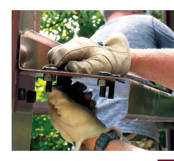
Engineered cees and zees **bolt together** with solid steel plates to give Centra<sup>™</sup> Series its strength.
