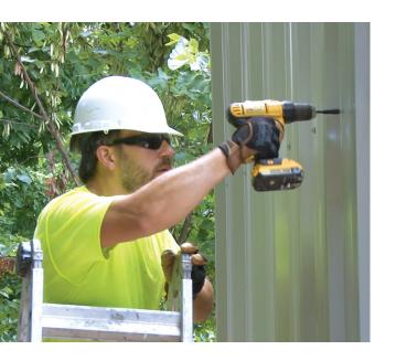
All you need is a **power drill** to attach the roof and wall panels.
